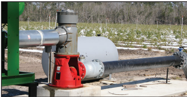
Miller Pump & Electric team up with NPC to grow blueberries in South Georgia. Pictured at left is a Hi-Pro head assembly with a combined right angle gear drive pumping 2000 GPM for frost protection and irrigation.
