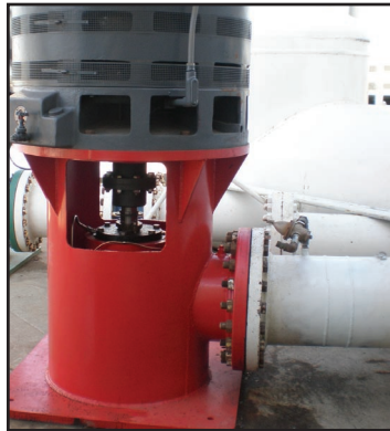
NPC H24XHC, designed to be more serviceable with the flange style coupling.
