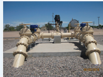
Figure 2 – Typical ASR Well Site
