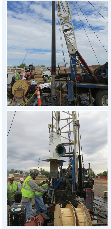
Figure 4 - Installation of VTP & Pump Column
